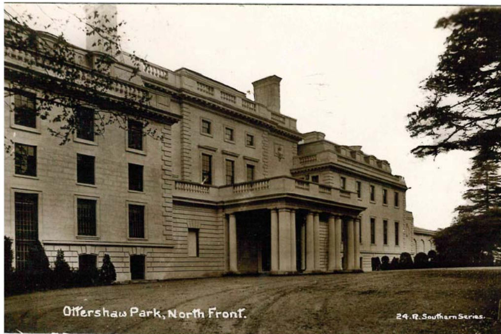
Southern Series 24R – the north front of the mansion
