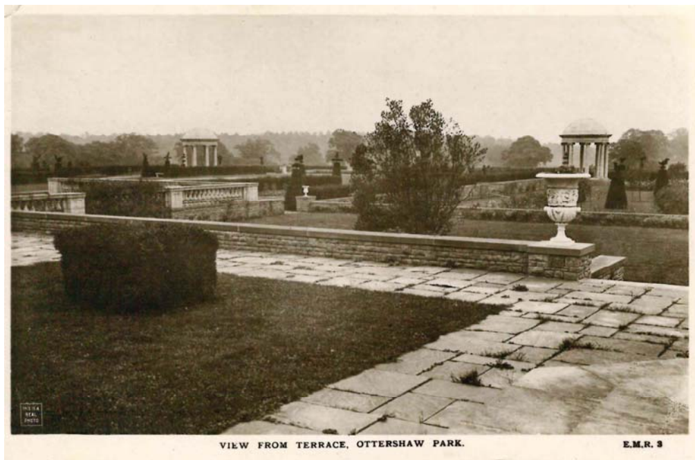
EMR 3 - A view from the terrace of the mansion during WWI
