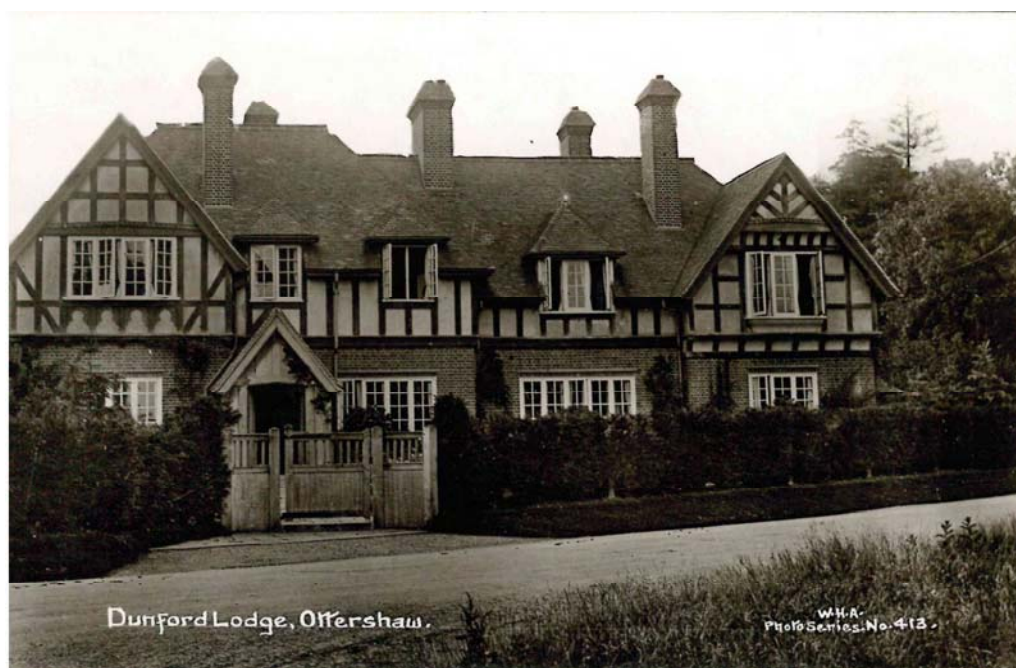
W.H.A. 413 – Dunford lodge (on Guildford Road) once the estate managers lodge
